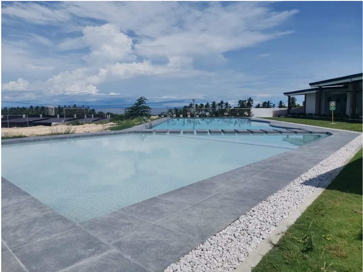
Latest construction updates of the Casa Mira South club house with a swimming pool.
